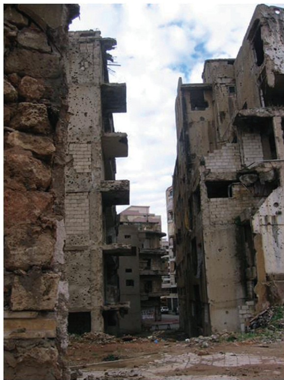
Figure 2. Two evacuated buildings in Hayy Madif Mar Michael Church neighborhood: an example of abandoned buildings where families settled who fled battles in South Lebanon in 1977. Many stayed there until 2004. Photo by author.
